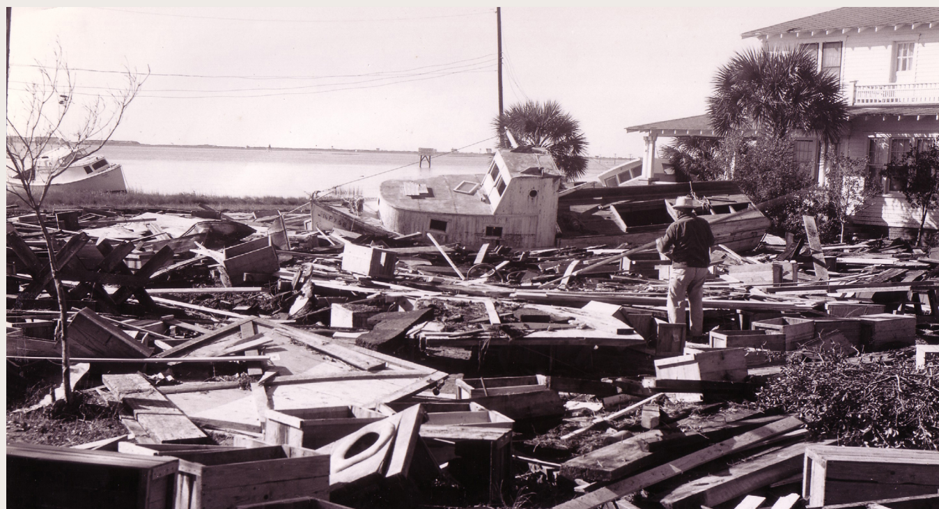
Destruction along the Southport waterfront in the wake of Hurricane Hazel.
